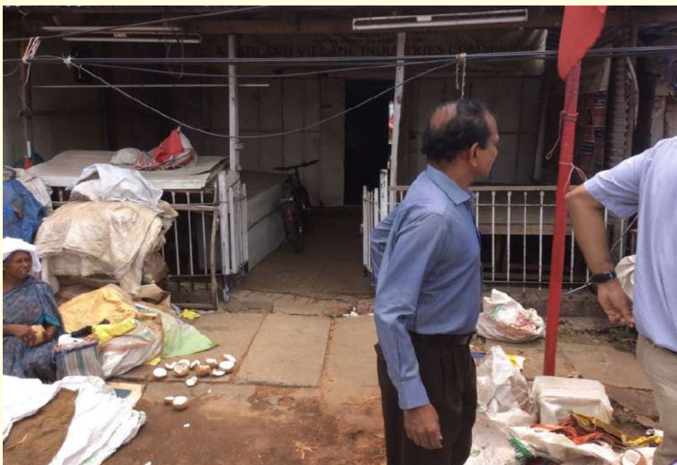
Figure 6 a shop on top of the drain
