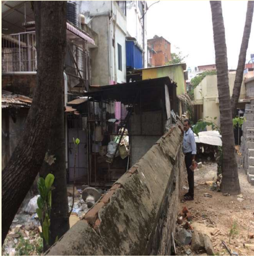
Figure 11 the green building is a generator room on top of drains
