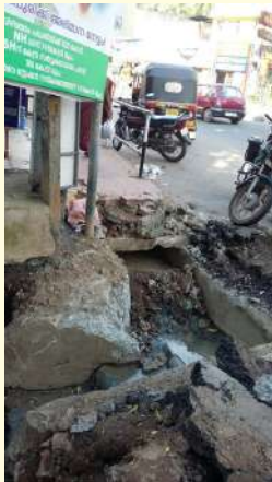
Figure 14 Drains chocked with deposited sand and debris
