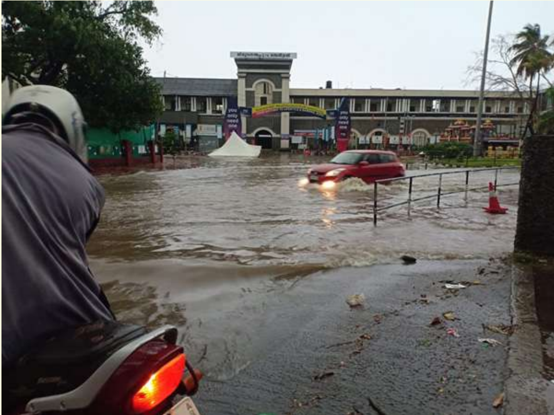
Figure 4 Thampanoor during floods
