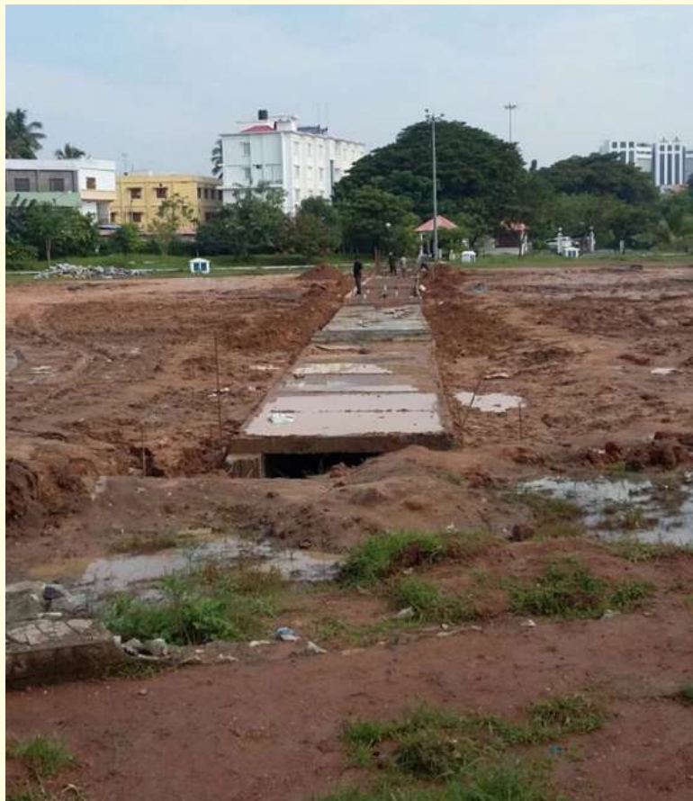
Figure 16 The overflow duct constructed to connect amayizhanchan and Thekkinikara canals
