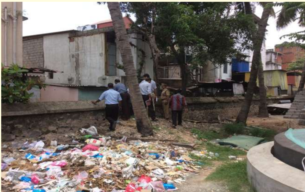
Figure 10 Buildings on top of the filled up drains
