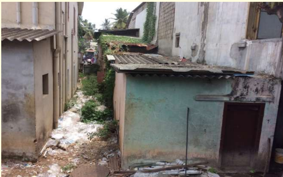
Figure 8 illegal construction on top of filled up drains
