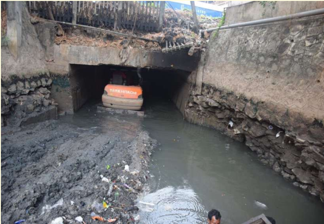
Figure 22 The excavator can pass through the box culvert under railway lines
